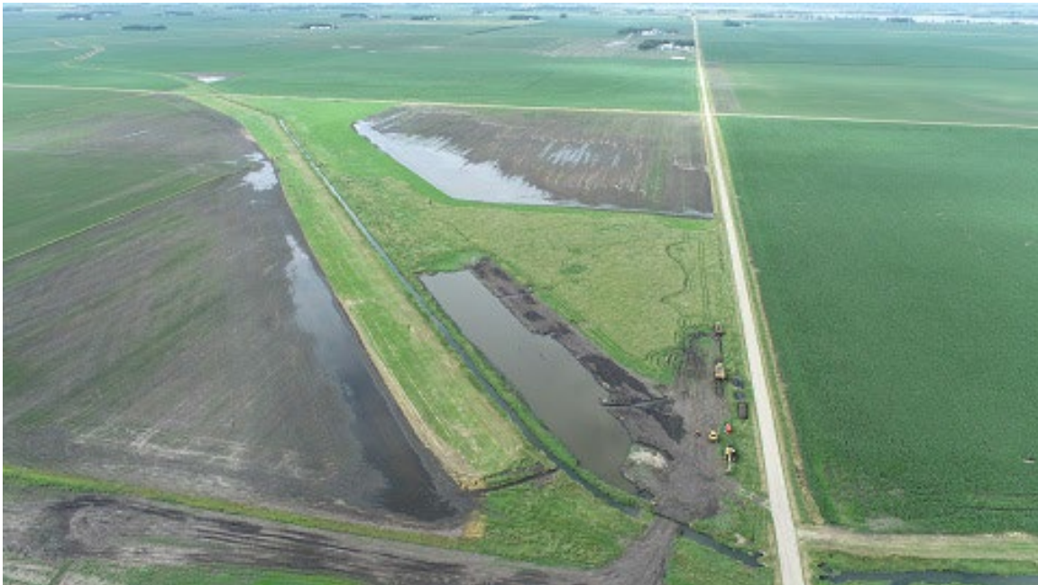
Figure 4 – This is a photo of a current County Ditch project. Improvements on this ditch system include this new holding pond to assist with water flow management into South Heron Lake outlet. We are also pursuing a conservation easement on this property.
